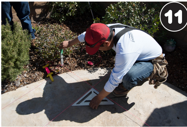
Adjusting the stake left to right to square the cover
