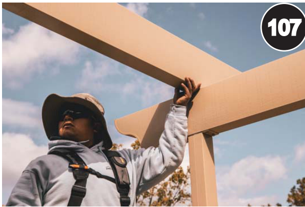
After the first rafter is installed they will square the rafter to the beam and ledger to confirm that the rafters are installed straight
